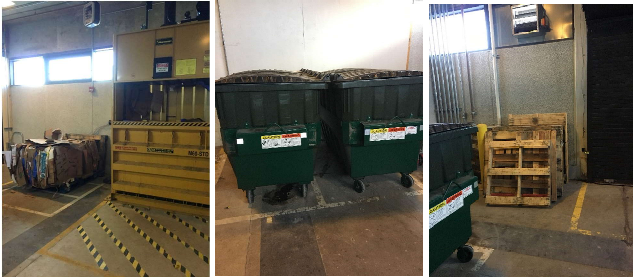
Figure 18: Airside waste and recycling area with a cardboard baler (left), two dumpsters for can and bottle recycling (center), and an area for pallets (right)
