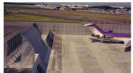
Everett/TRAMCO (USA) Project Highlight: "L" shaped facility.
