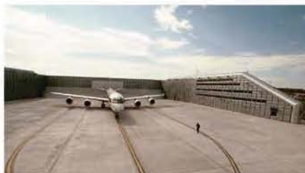
Milwaukee (USA) Project Highlight: Facility was installed directly on existing aircraft pavement.
