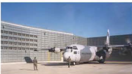
Chicago O'Hare (USA) Project Highlight: First installation of BDI's Stable Flow™ system.
