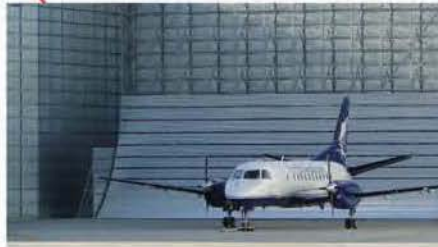
Vancouver (Canada) Project Highlight: LED signage on cladding.
