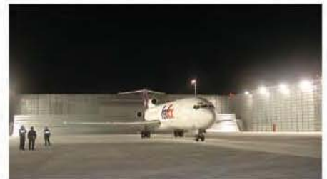
Oakland (USA) Project Highlight: Aircraft up to B747 can perform run-ups in GRE.
