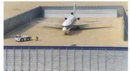
Portsmouth (USA) Project Highlight: Last non-vented GRE built by BDI.
