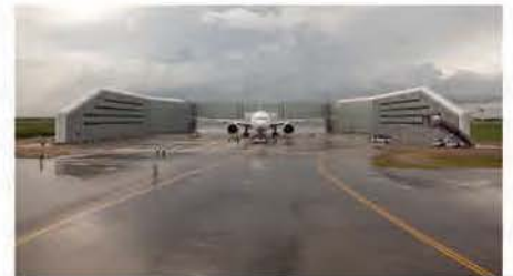
Bangkok (Thailand) Project Highlight: Accommodates A380 and MD-11.
