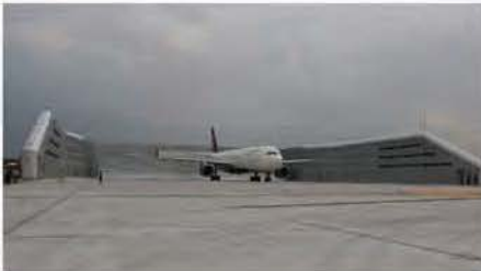
Detroit (USA) Project Highlight: Anti-radar cladding on exterior.
