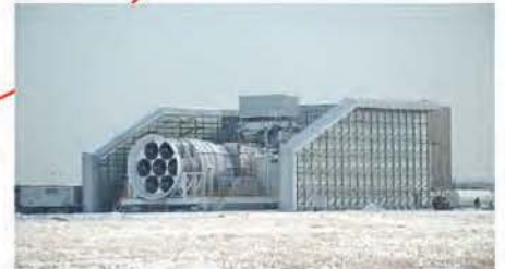
Winnipeg/GE (Canada) Project Highlight: Engine ice test facility with Augmentor & exhaust stack.
