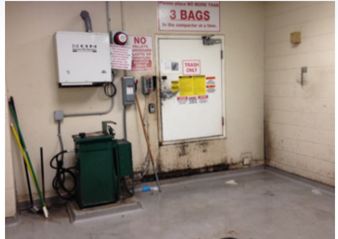
FIGURE 7 SOLID WASTE COMPACTORS AT MKE LANDSIDE TERMINAL (TOP) AND AIRSIDE (BOTTOM)
