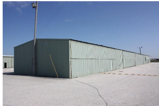
Figure 3.7. T-hangar E/F Source: Hanson Professional Services Inc., May 2017.
