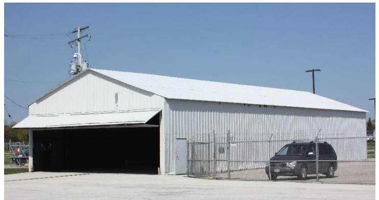
Figure 3.16. Schwartzburg Hangar Source: Hanson Professional Services Inc., 2017.
