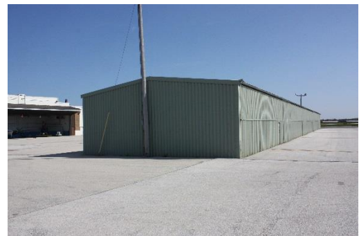
Figure 3.5. T-hangar A/B Source: Hanson Professional Services Inc., May 2017
