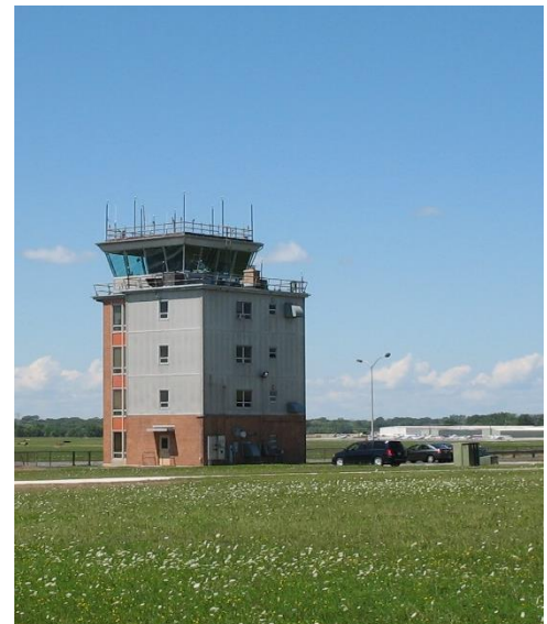
Figure 3.19. Airport Traffic Control Tower
