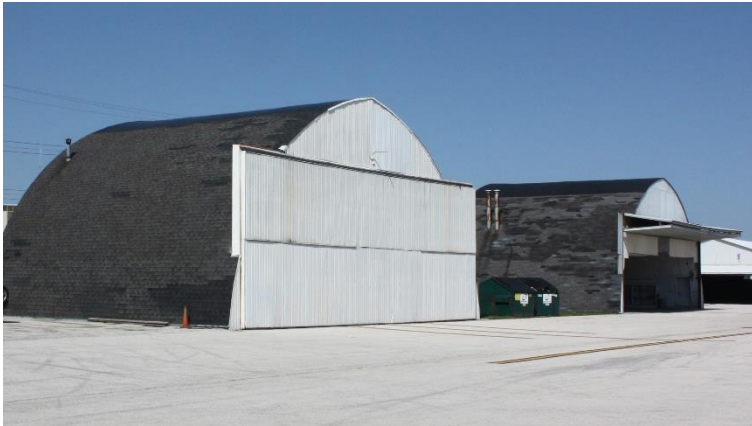
Figure 3.14. Middle and East Quonset Hut Source: Hanson Professional Services Inc., May 2017.
