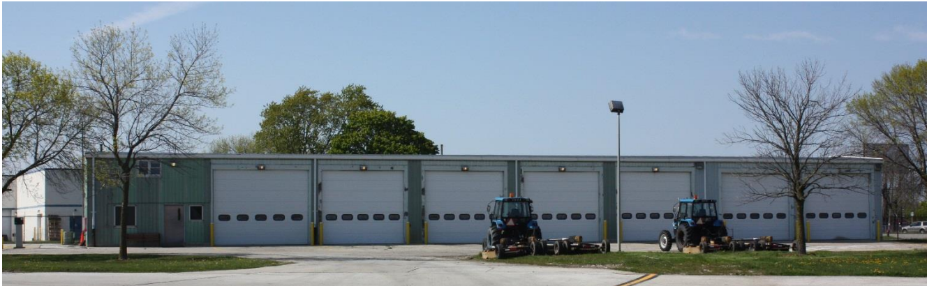
Figure 3.17. County Maintenance Garage Source: Hanson Professional Services Inc., May 2017
