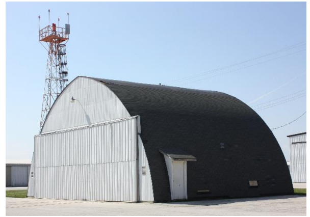
Figure 3.15. West Quonset Hut Source: Hanson Professional Services Inc., May 2017.
